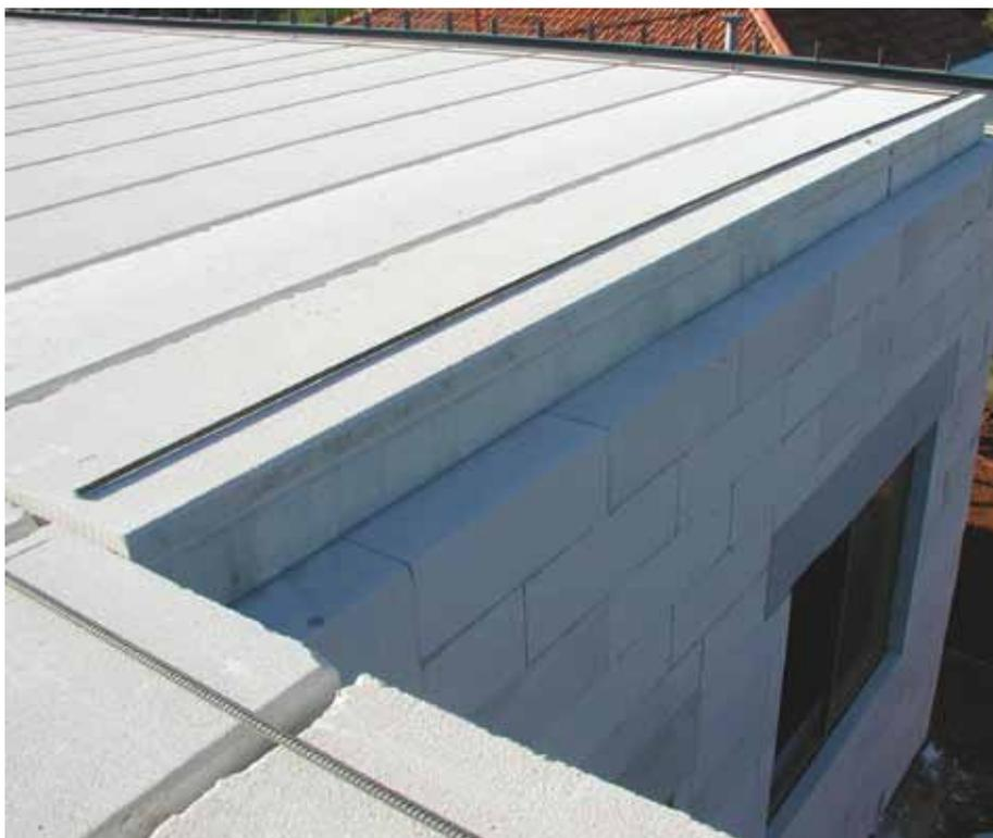
**Image 7.3.3: Installing Floor Panels**
