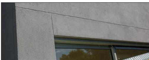
Figure 3.4.1 Neat finish of horizontal joints
